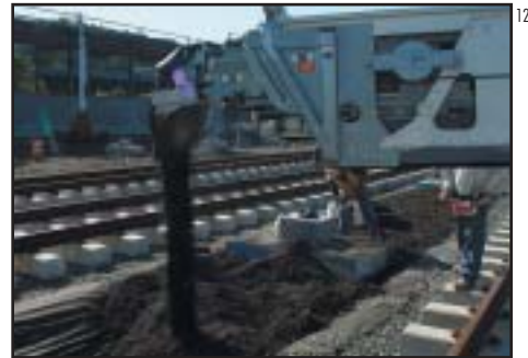
Soil backfill
