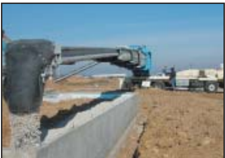
Drainage stone - foundation
