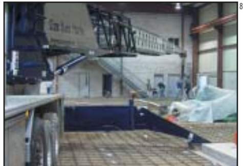
Inside slab - low clearance
