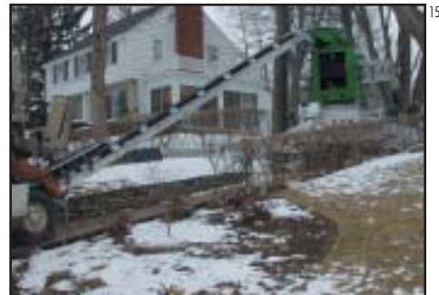
Difficult residential setup
