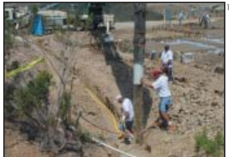
Utility trench backfill
