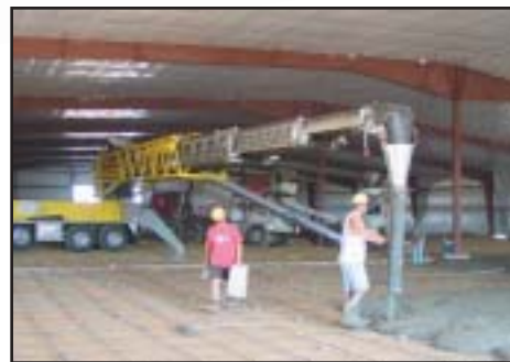
Slab on foam insulation
