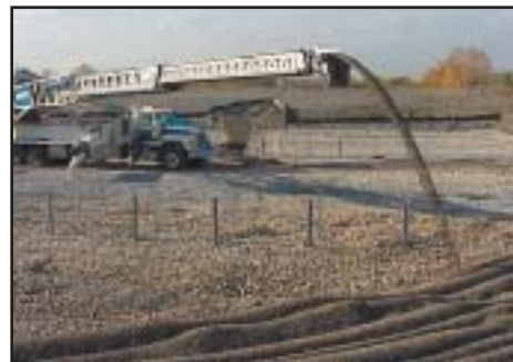
Aggregate on settling basin
