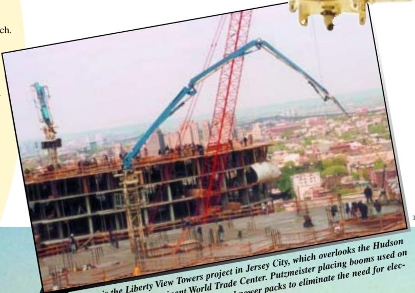
Above is the Liberty View Towers project in Jersey City, which overlooks the Hudson River at the once prominent World Trade Center. Putzmeister placing booms used on this job feature specially-designed diesel power packs to eliminate the need for electrical hook ups and save the contractor money.
