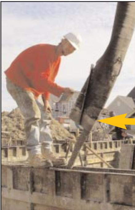
**7.** Curving the endhose allows the mix to remix itself before it flows into the wall forms. It also slows down the free fall effect that may occur after the material leaves the belt.
