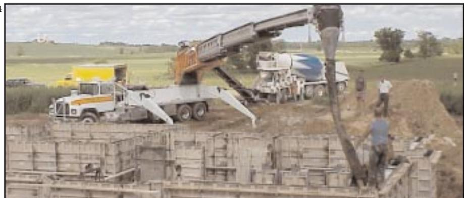
**10.** Stand between the feeder and the main boom to correctly control the flow of material from the ready-mix truck through the belt to the pour.
