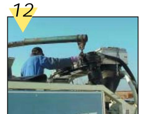
Lift the drive unit out through the top of the boom truss.
