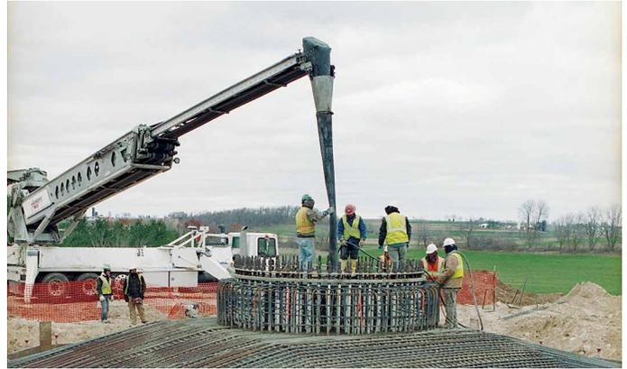
Rather than using a pump, Sanderfoot Wind placed material with two Putzmeister Telebelt® TB 110 telescopic belt conveyors (the company owns four).
