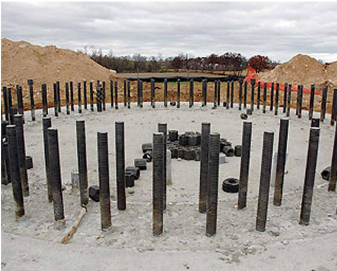
123 Cedar Ridge turbines will bear on two rings of 1½-in.-diameter threaded tower anchor bolts, ranging in number from 120 to 144, embedded nearly 8 ft. deep.
