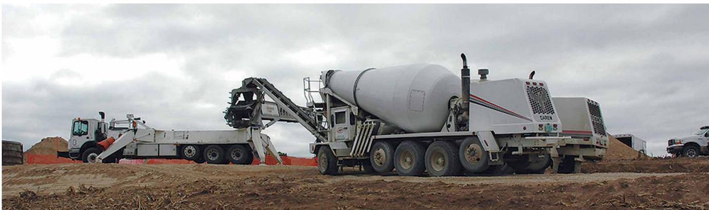
At the 41-turbine Cedar Ridge wind farm job site, crews raced against time and the elements with only 22 days to pour pedestals before cold temperatures threatened to freeze portable plant water supplies. Lead contractor Sanderfoot Wind deployed two Putzmeister Telebelt conveyors, making certain that they were constantly charged with material and never turning them off during a shift. As a result, two or three pedestals were finished per day.
