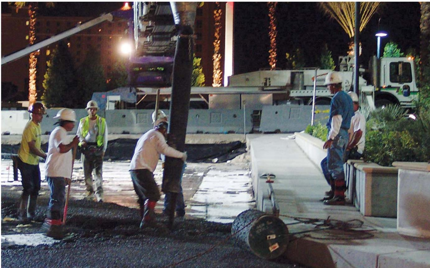
After placing the last third of the pervious concrete, Steve Heimark says this type of concrete could be a good thing for the Las Vegas area. Three separate pervious concrete placements occurred to complete the driveway for the second tower of the MGM Residence Tower and totaled at 325 cubic yards.
