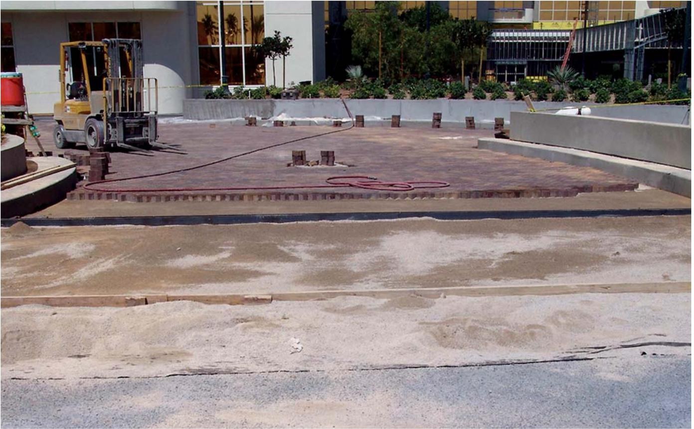
The last step of the driveway construction; two-inch brick pavers are placed on top of the two inches of sand for the second tower driveway of the MGM Residence Towers.
