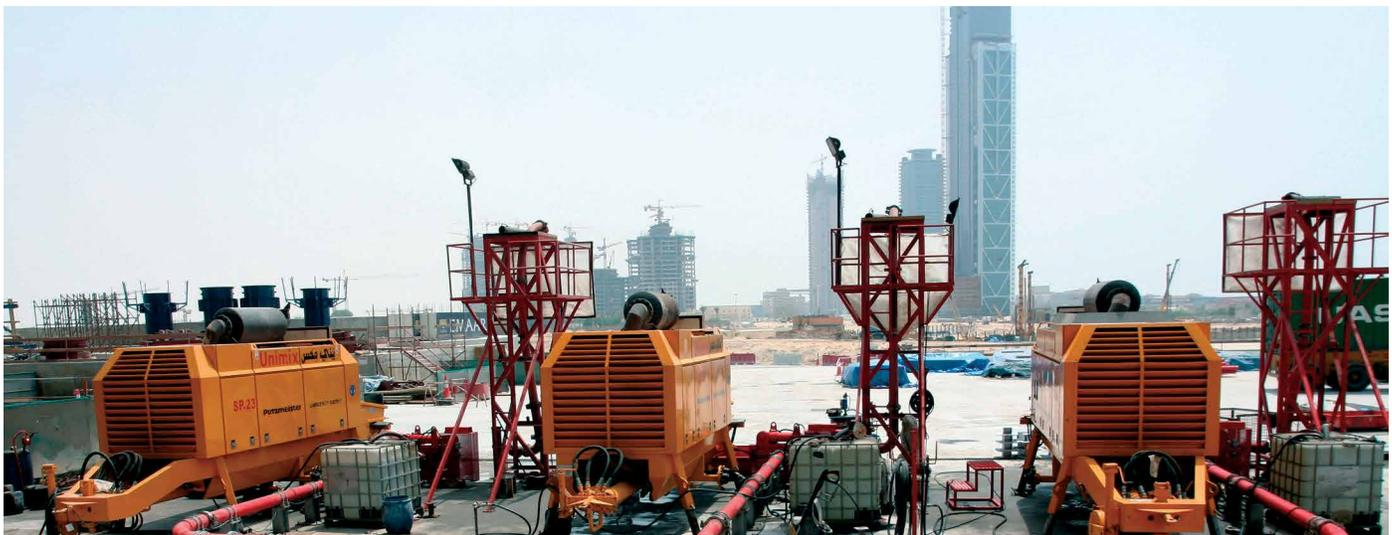
Three BSA 14000 trailer pumps were combined to create one pump station for this project.
