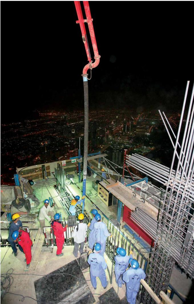
6 Three MX 28-4 T and one MX 32-4 T placing booms, in addition to various truck-mounted boom pumps, were on site to place the concrete.
