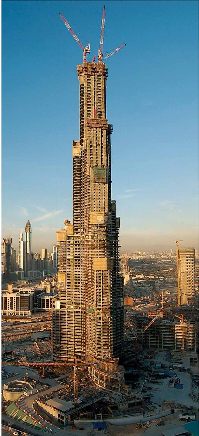
7 Throughout the entire project, only high compressive strength concrete mixtures were used and pours were only done at night because of hot temperatures during the day.
