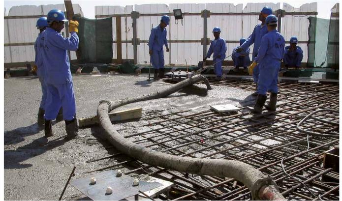
The pumping station pumped approximately 5,826,920 cu. ft. (165,000m<sup>3</sup>) of high-strength concrete during the 32 months of operation.
