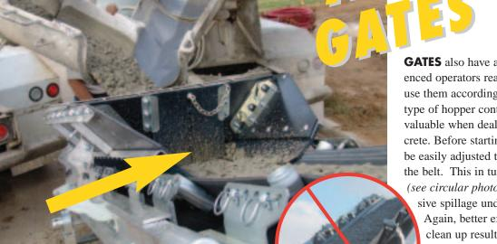
**GATES** also have a purpose and experienced operators realize their value and use them accordingly. The gate – a type of hopper control – is especially valuable when dealing with wet concrete. Before starting the job, they can be easily adjusted to avoid over-filling the belt. This in turn prevents waves (see circular photo) and avoids excessional starting the best of the bes
