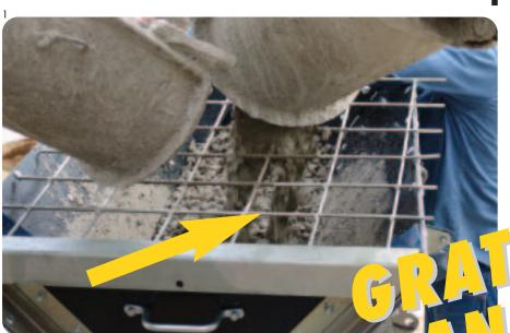
**GRATES** have a purpose, and wise operators use them for enhanced safety, increased efficiency and reduced clean up. The grates prevent large objects – rocks, ice balls, and even hard hats – from going up the belt and plugging the transfer and reducer. This can cause delays on the job and create a mess to clean up afterwards. Basically, the message is **USE YOUR GRATES!**
