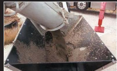
For a belt, the hopper is for guiding material (see above). For a boom pump, the hopper is for filling.
