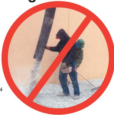
Above: Incorrect positioning especially with the operator at the end hose.
