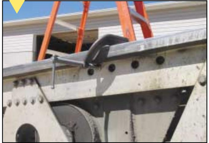
If you need to move a section to the side in order to insert a block, a C-clamp works well for moving and holding the section in the desired position.
