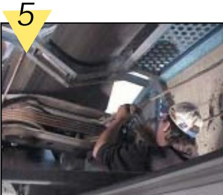
5 Remove the cable attachment at the telescope drive (TB 105) or spring tensioner (TB 130). Remove the cable clamps and thimble and cut the cable, if necessary to make sure it is straight. If the existing cable has a swaged socket, cut it off.
