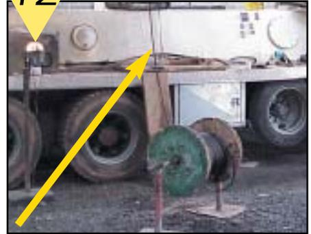
This shows the cables joined and ready to pull (at arrow).
