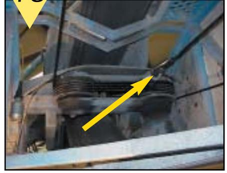
Stop the pulling operation when the swaged socket can be connected to the anchor (TB 105) or spring tensioner (TB 130). **Shut the unit off to make the connection.**
