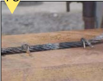
Match the end of the new cable with the end you removed from the anchor point.
