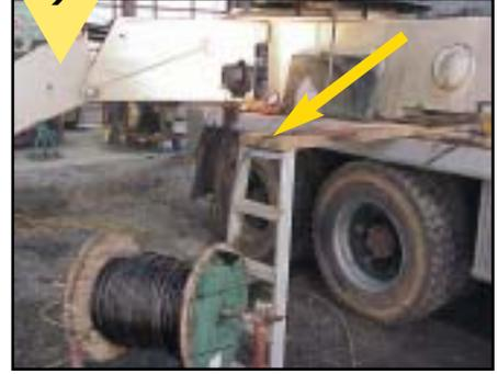
Cables supplied by Putzmeister have a swaged socket on one end. Leave the socket wired to the side of the cable reel, as shipped. Place the reel on stands, with the cable running from the bottom of the reel toward the truck.
