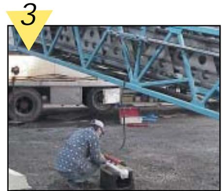
3 Connect the tensioning jack to the cable tensioning cylinder.
